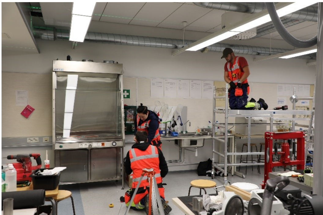
FIGURE 13. Installation of air-conditioned cabinet (Brask 2021)
