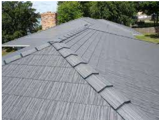
Figure 5. Steel roof (Abcseamless, 2020)
