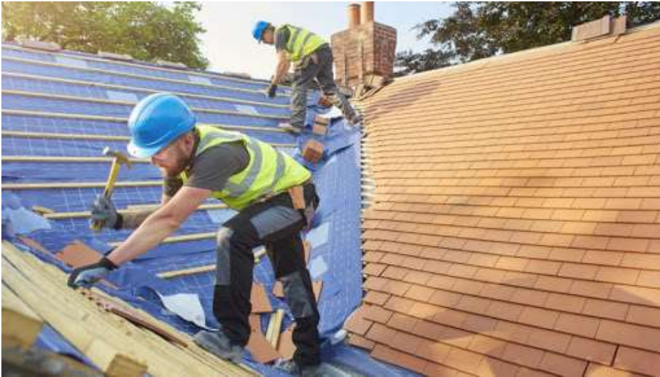
Figure 1. Roof manual installation (Next Insurance , 2020)
