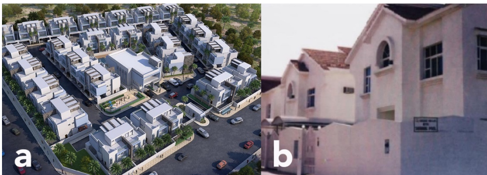
Fig 6 a) high perspective of muraikh residential compound in Doha city (Ibrahimjaidah, 2020). b) Private villa housing in Doha city (Alshawish, 2016)
