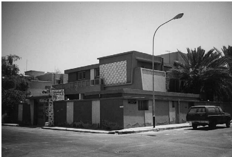
Fig 5 window screening with higher parapet as a classic privacy technique in houses having higher floors (Saleh, 2002)
