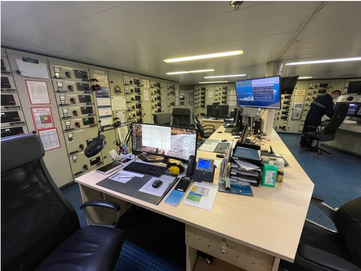
Figure 16 Astoria Grande Engine Control Room (Author, 2022)
