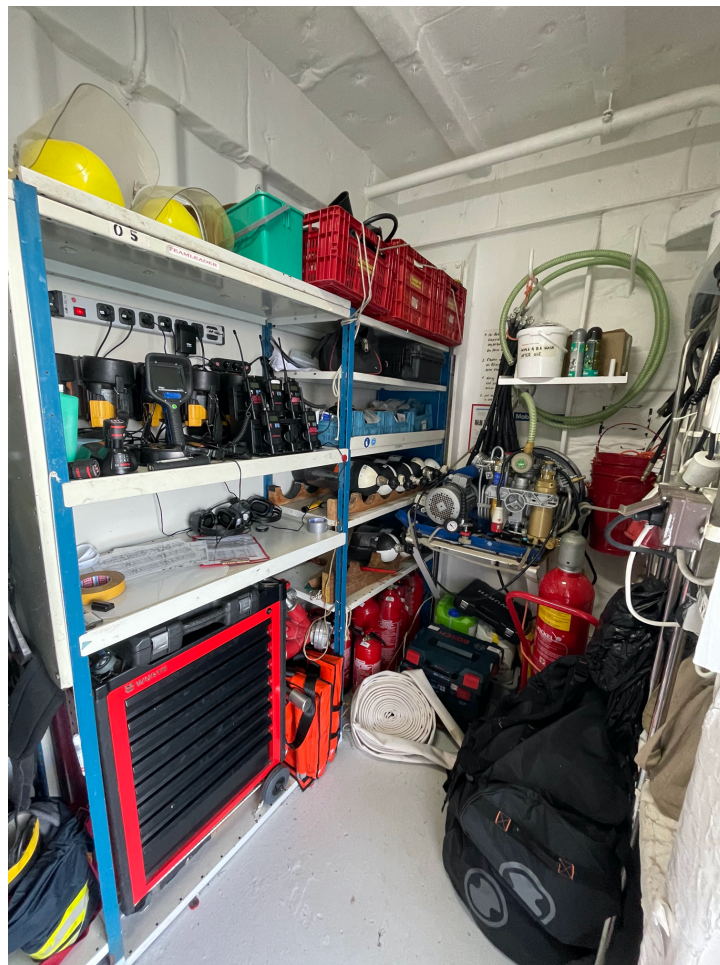
Figure 24 Fire locker equipment (Alo Kask, 2022)
