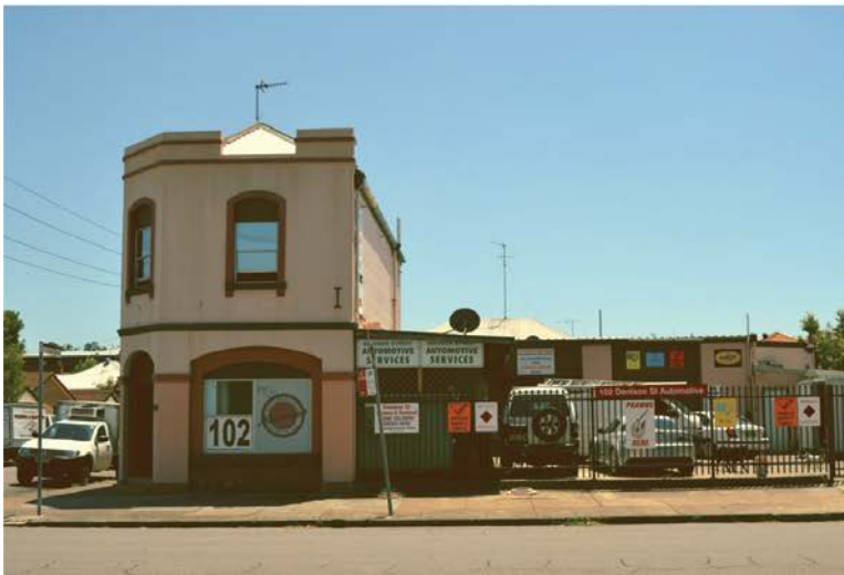
Picture 1. Some mechanical companies in Newcastle area.
