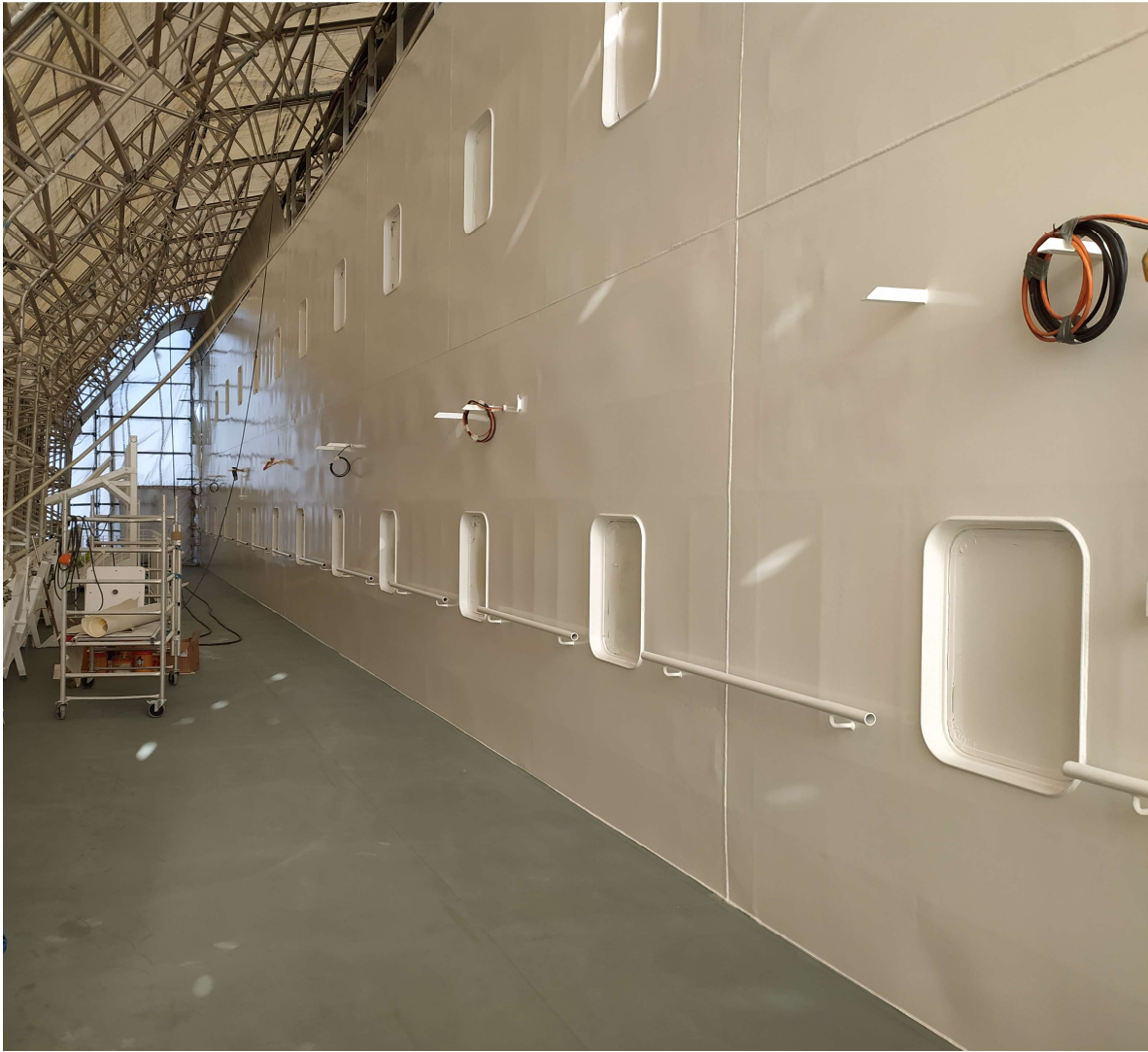
Figure 12: Top-coated outer bulkhead. Deck level is sprayed with zinc primer.
