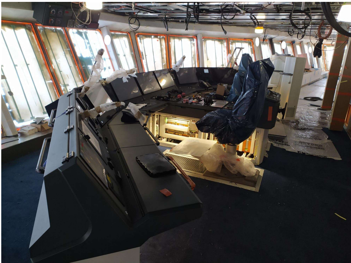
Figure 22: Navigational bridge cockpit under construction, taking shape.
