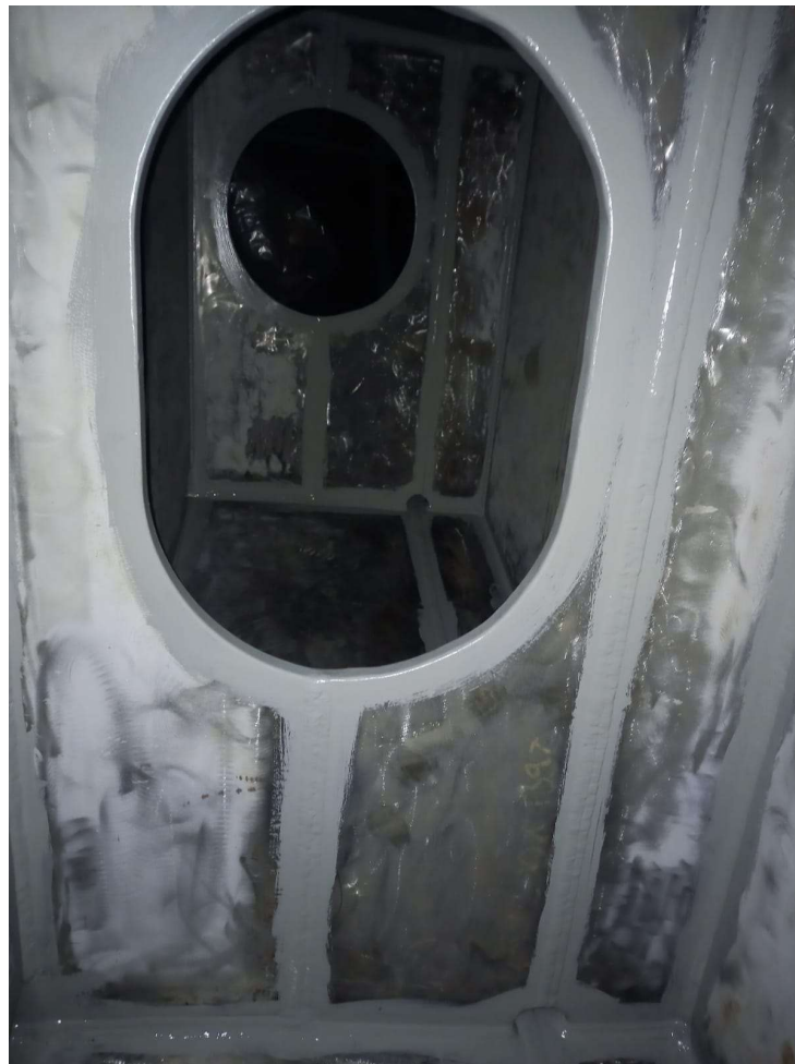
Figure 10: Example of stripe coat. The corners, edges and welds are pre-coated prior spraying.
