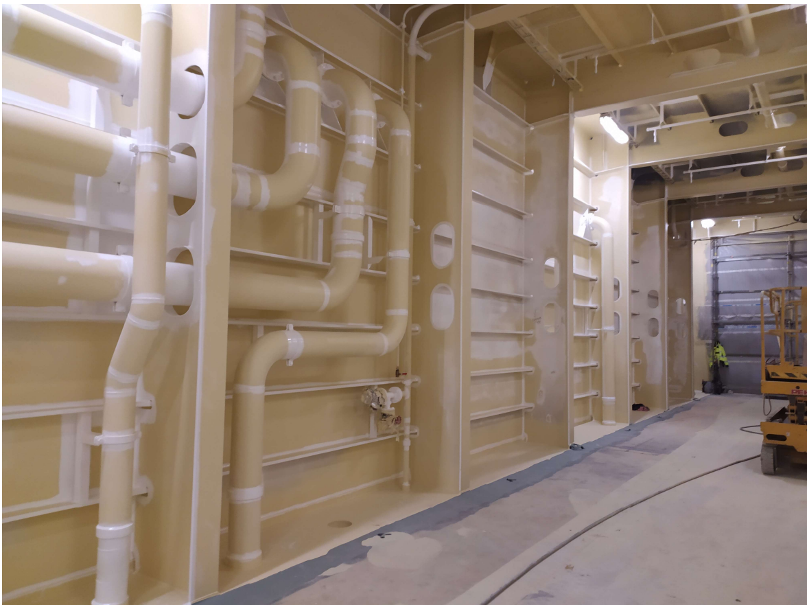
Figure 11: Primer covered bulkhead on cargo area. Top layer stripe coat also applied.
