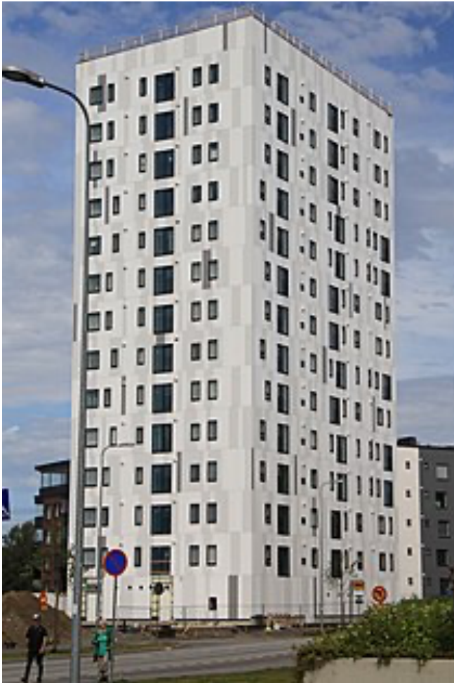
Figure 3. Jonsulight house. This photo is from Puuinfo OY
