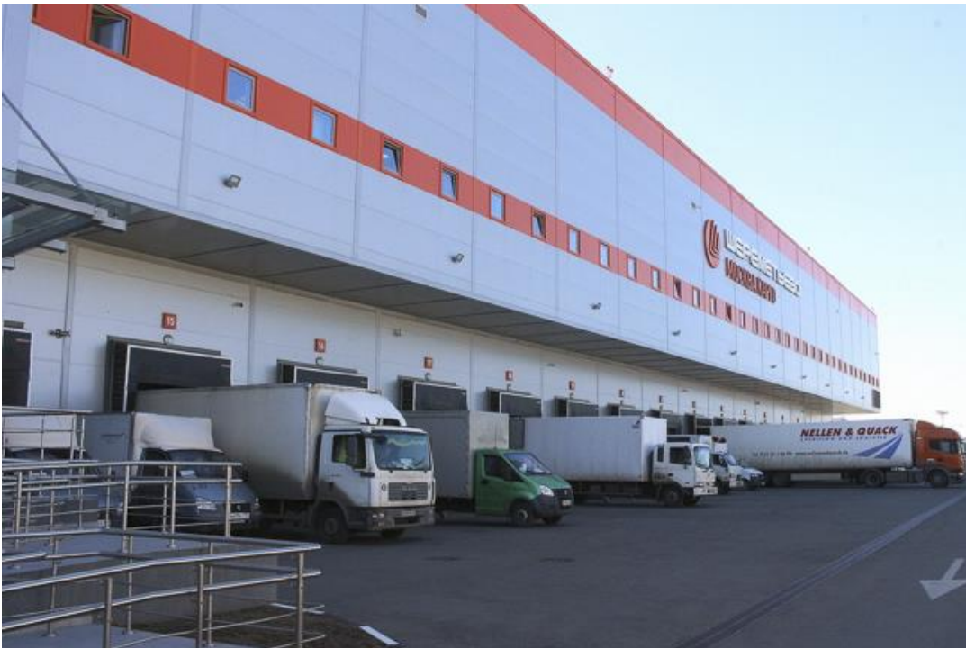
Figure 1. Moscow Cargo terminal
