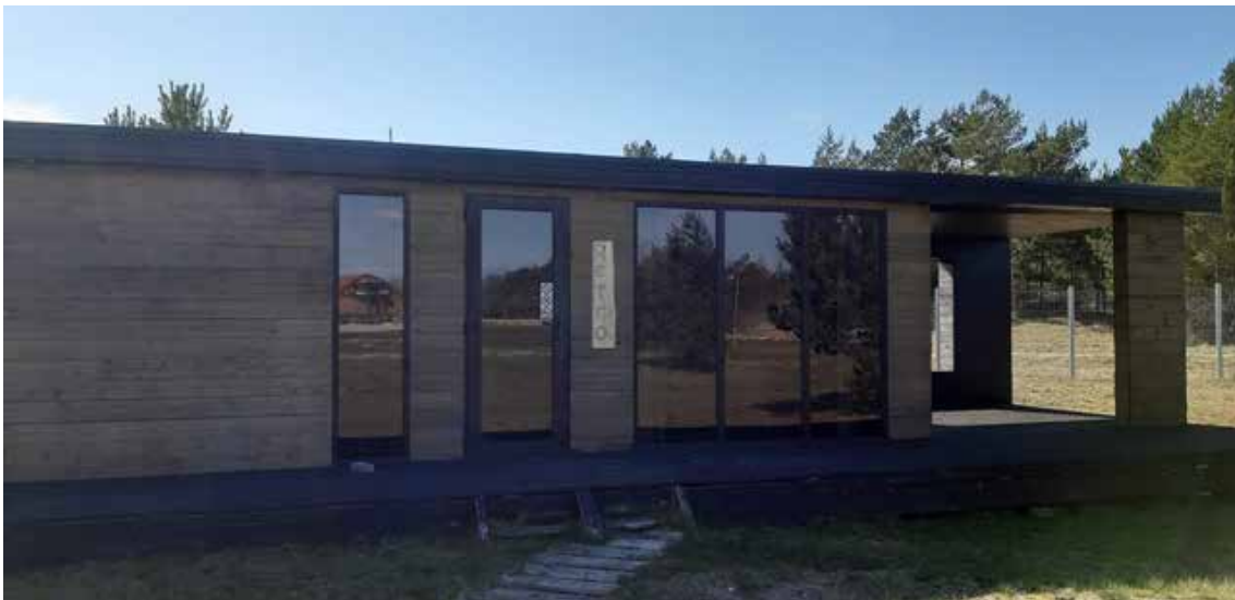
Picture 3. One of the four Pavilosta Marinas separate holiday houses.
