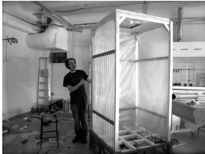
Figure 10. Construction of the ShowerMagic ‘demonstration’ stall in the Environmental Engineering Lab. The frame was made from wood beams and polycarbonate roof sheeting. A bilge pump was used to collect and pump water to the showerhead, which was made from the same materials as the stall walls. The front door and floor are still missing.
