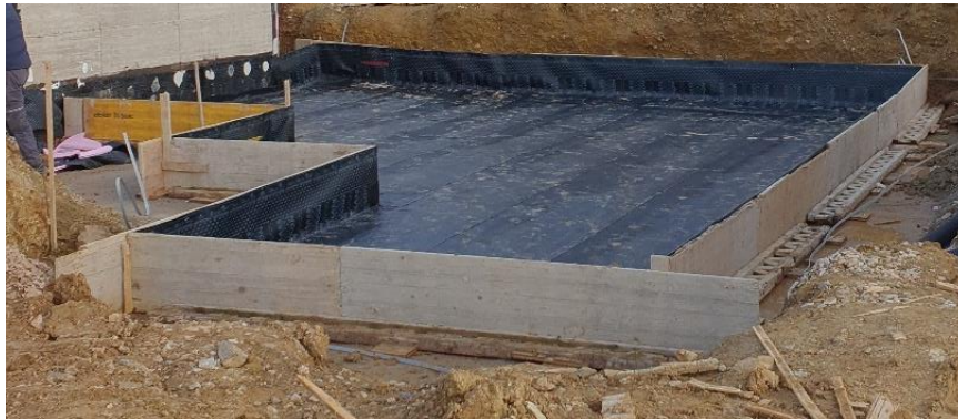
Figure 3 4 mm waterproof barrier placed to protect slab foundation from being damaged
