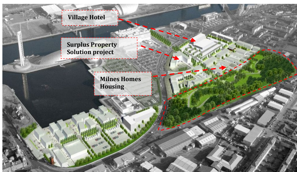
Figure 16: Aerial view of housing projects in Old Festival Park (Source: Pacific Quay Project)
