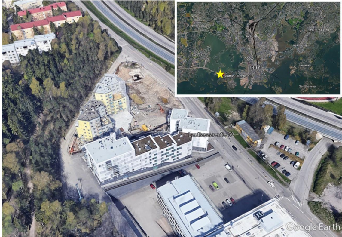
Figure 2. Green roof at Lauttasaarentie 52 (Google Earth, 2022)
