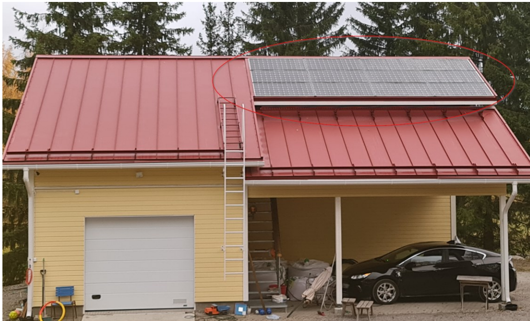
Figure 21. The panels on the roof of garage (Niskala 2022)
