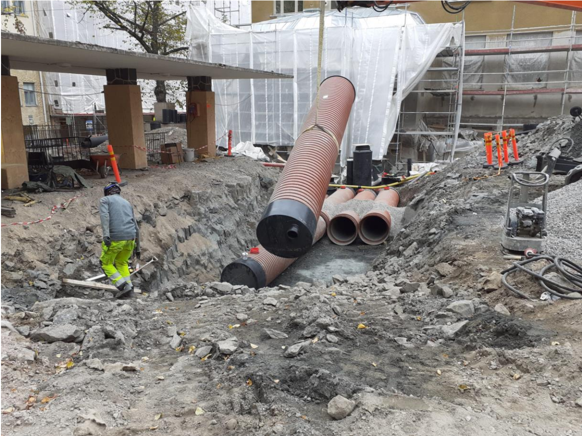
Image 17. Retention tanks being installed in Helsinki. (Andrew Atkinson 2022)
