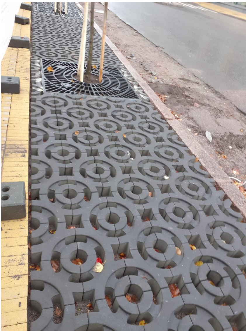
Image 12. Pervious paving installed in Tuusula. (Andrew Atkinson 2020)
