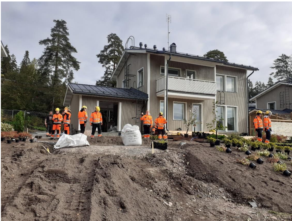
Image 10. Pellas ready for planting. (Andrew Atkinson 2021)
