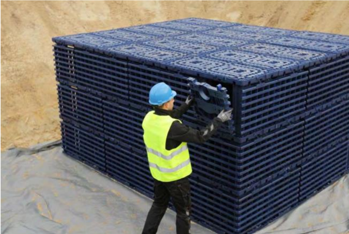
Image 14. Installing the Q-Bic system. (Wavin 2022)
