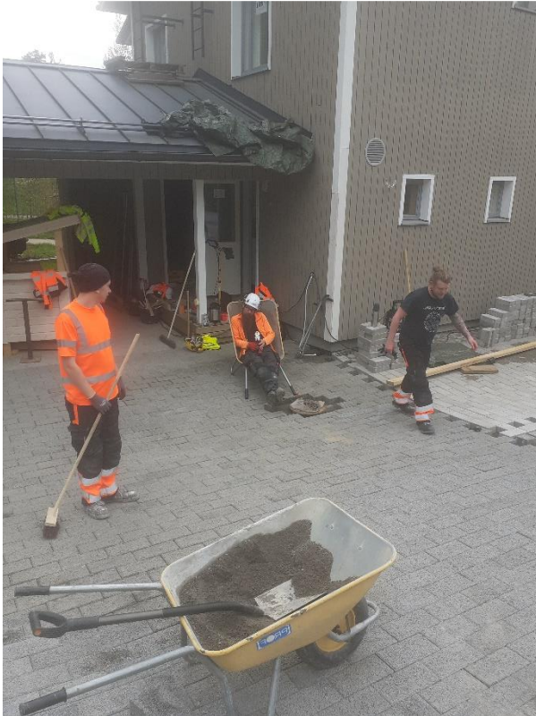
Image 9. HB-Betoni's pervious concrete 'Hulekivi' installed at Pellas. (Andrew Atkinson 2021)
