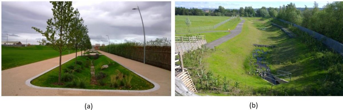
Figure 17: Existing SUDS in Dalmarnock (a) Raingardens in Colvend street (b) South Dalmarnock Regional Pond
