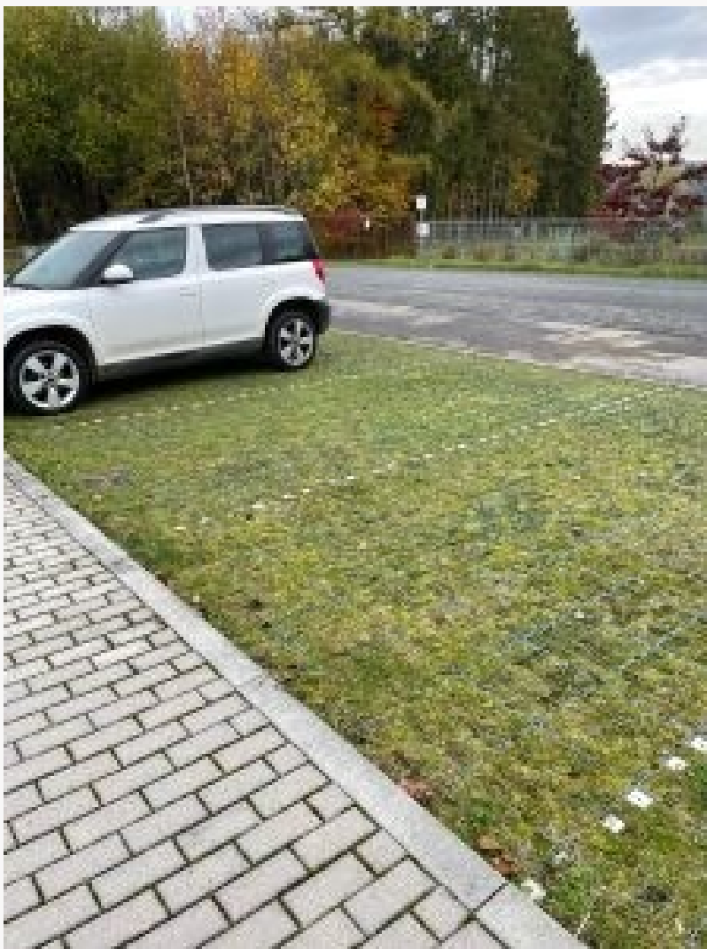
Figure 1: Phyto-Parking in allows for more sustainable stormwater management in areas where no additional land is available and no excavation is allowed, for example due to planning restrictions to protect heritage assets. (Joe Perry, 2022)
