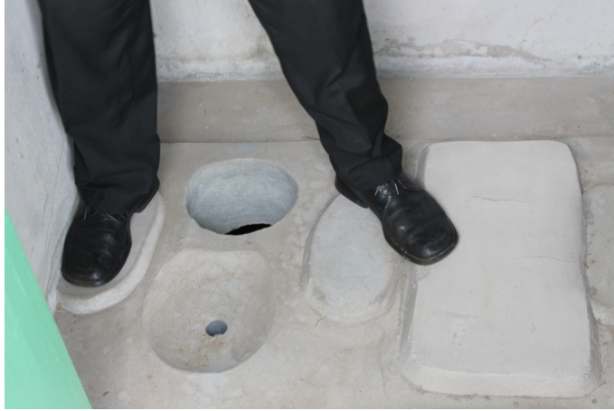
FIGURE 7. Urine diverting squatting pan and closed squatting pan
