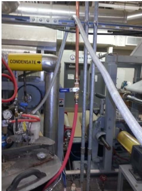
FIGURE 14. New hot water line
