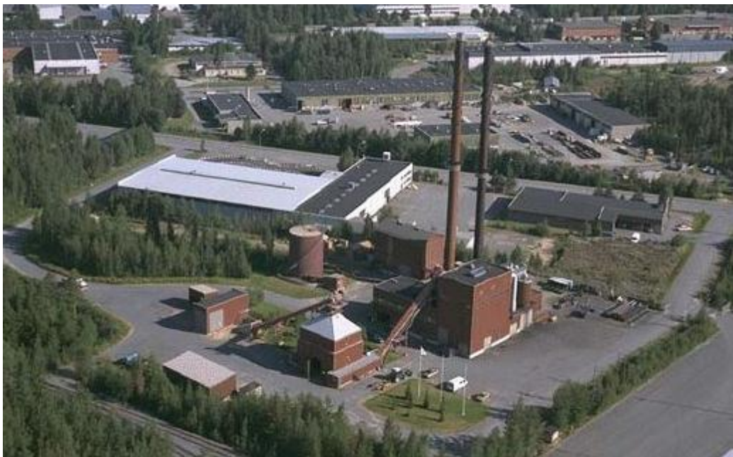
Figure 1. Seinäjoen Energia Oy's heat plant in Kapernaumi (Masinotek 2013)
