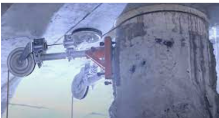
Figure 25. Example of diamond saw wire installation for column cut.
