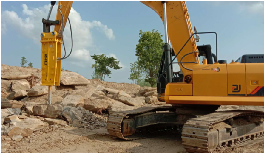
Figure 9. Excavator with pneumatic breaker attachment under work.
