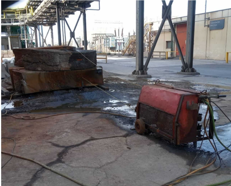
Figure 5. Diamond wire saw equipment under work. (Aracorte, n.d.)
