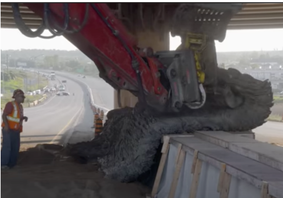
Figure 29. Mechanical installation of protection mats over road barriers.
