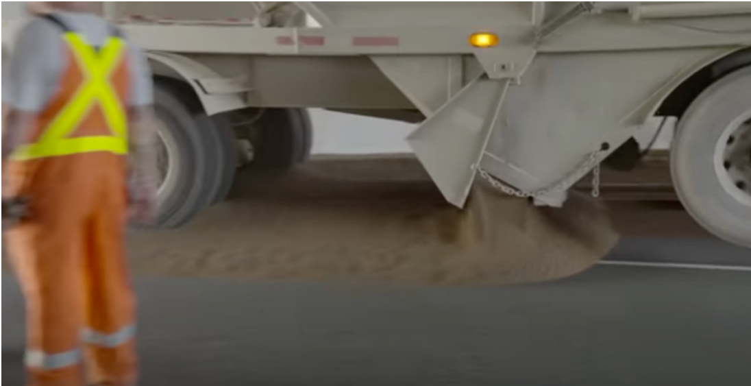
Figure 28. Example of spreading procedure of sand.
