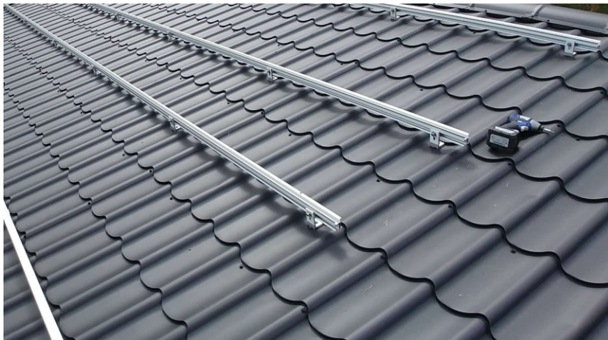
Figure 3. Roof mounting and rails for solar panel installation
