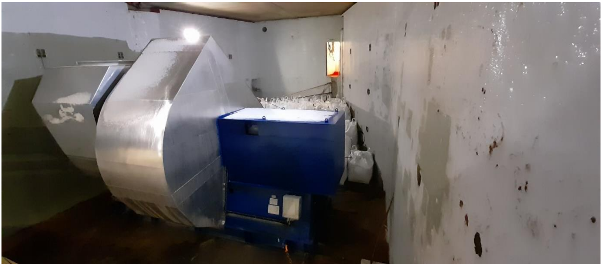
Figure 35: Fan is welded on deck, secured with chains and speed lashes.
