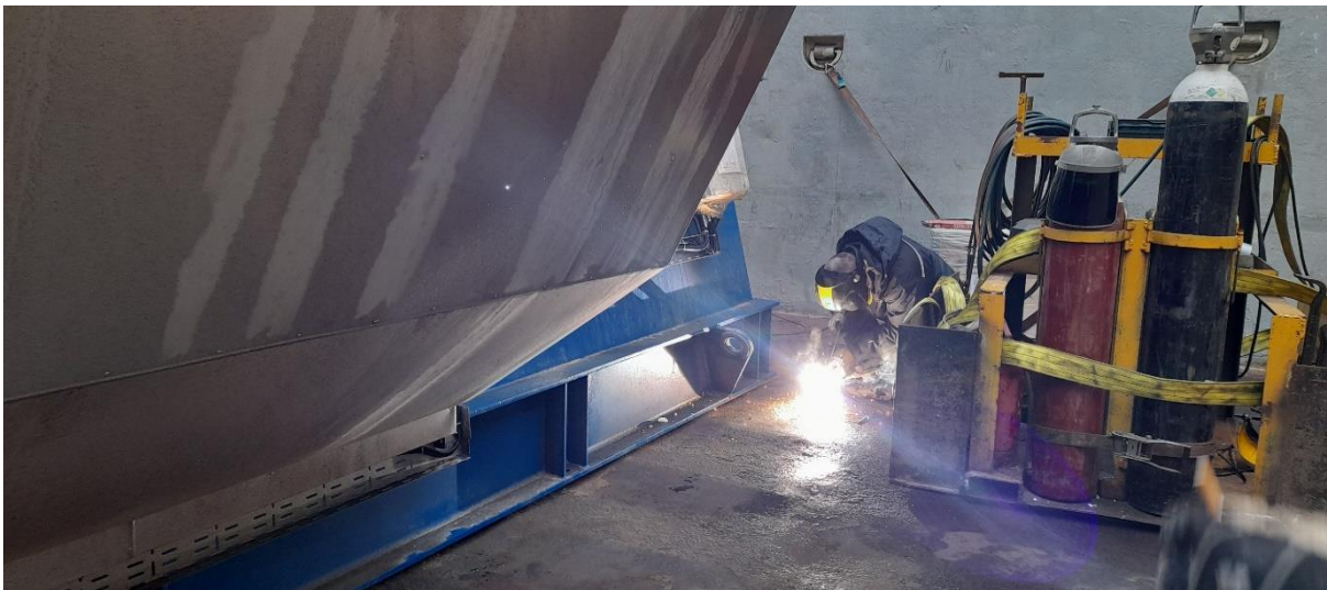
Figure 33: The process of welding the special project cargo Fan onto deck.
