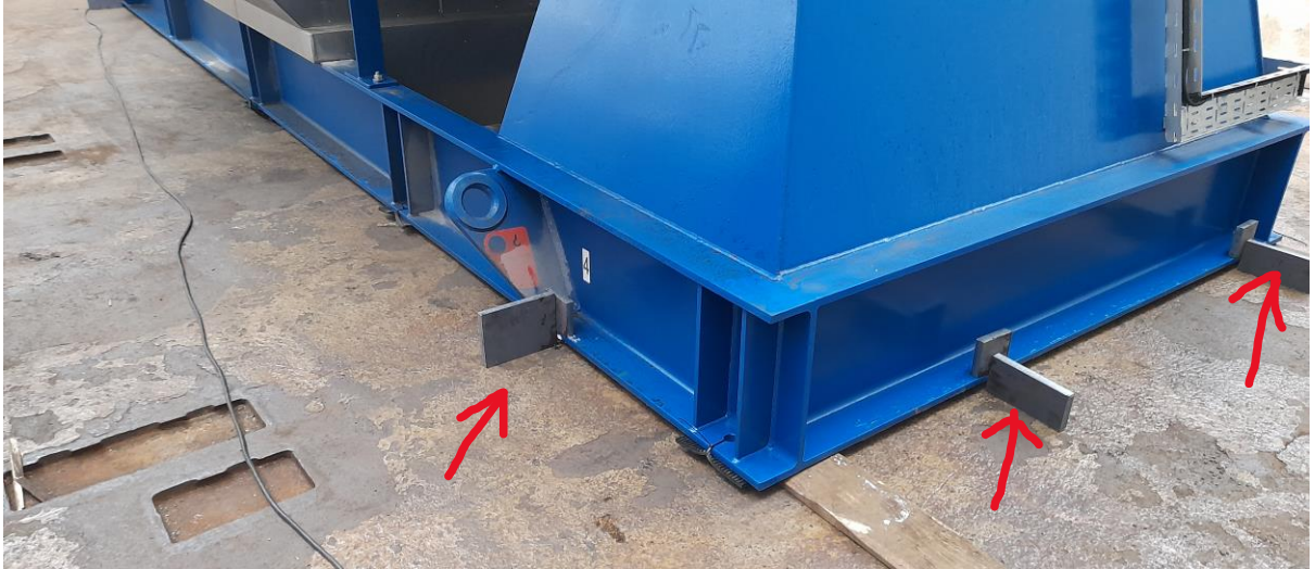
Figure 34: The Stoppers that will be welded to deck.
