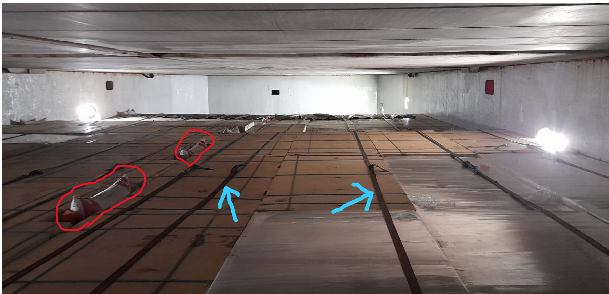
Figure 15: View from the top of the plywood on the tween deck where we can see the airbags.
