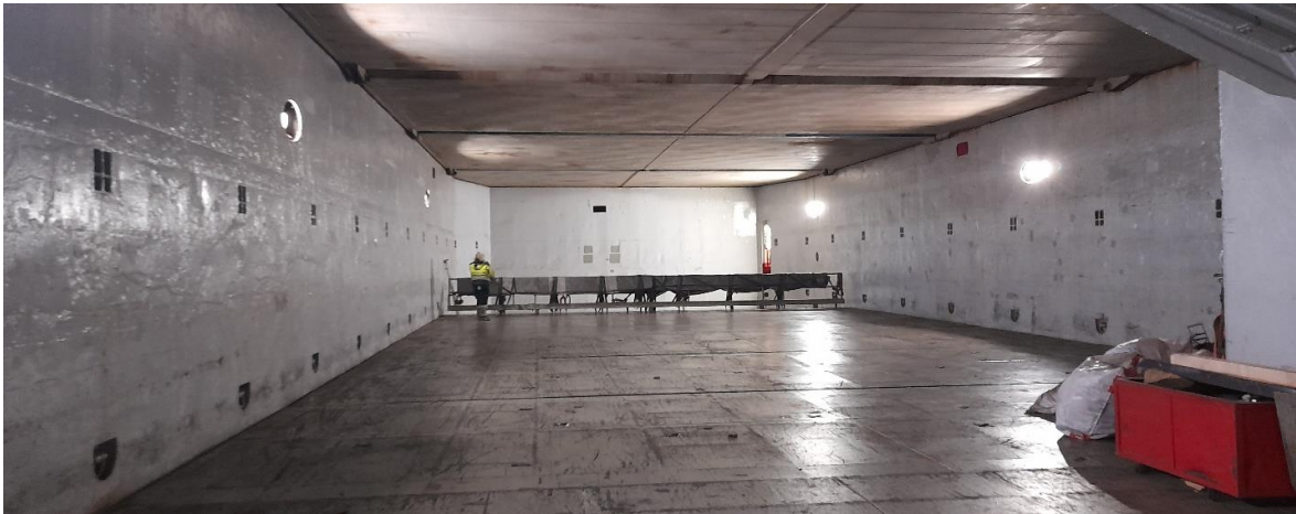
Figure 7: Preparation of the tween deck for plywood.
