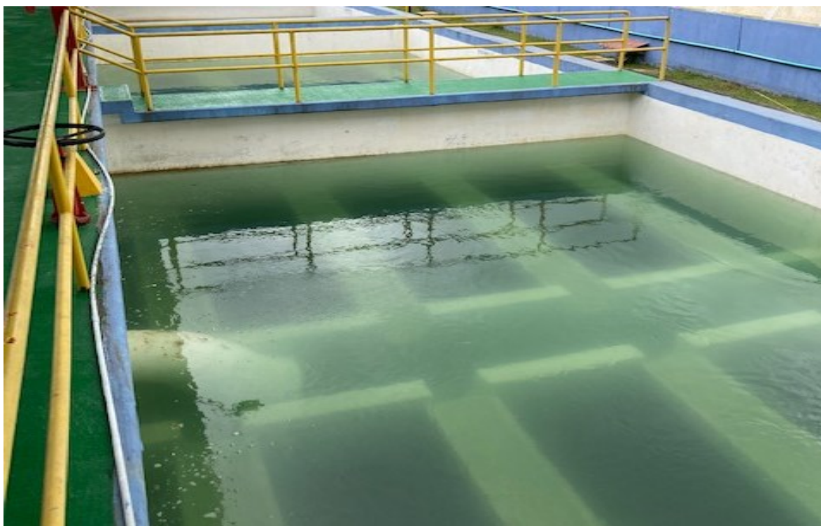
FIGURE 4. Sand filtration basin at AyA Tres Ríos water treatment plant (Hoffrén 2023, CC BY-NC)
