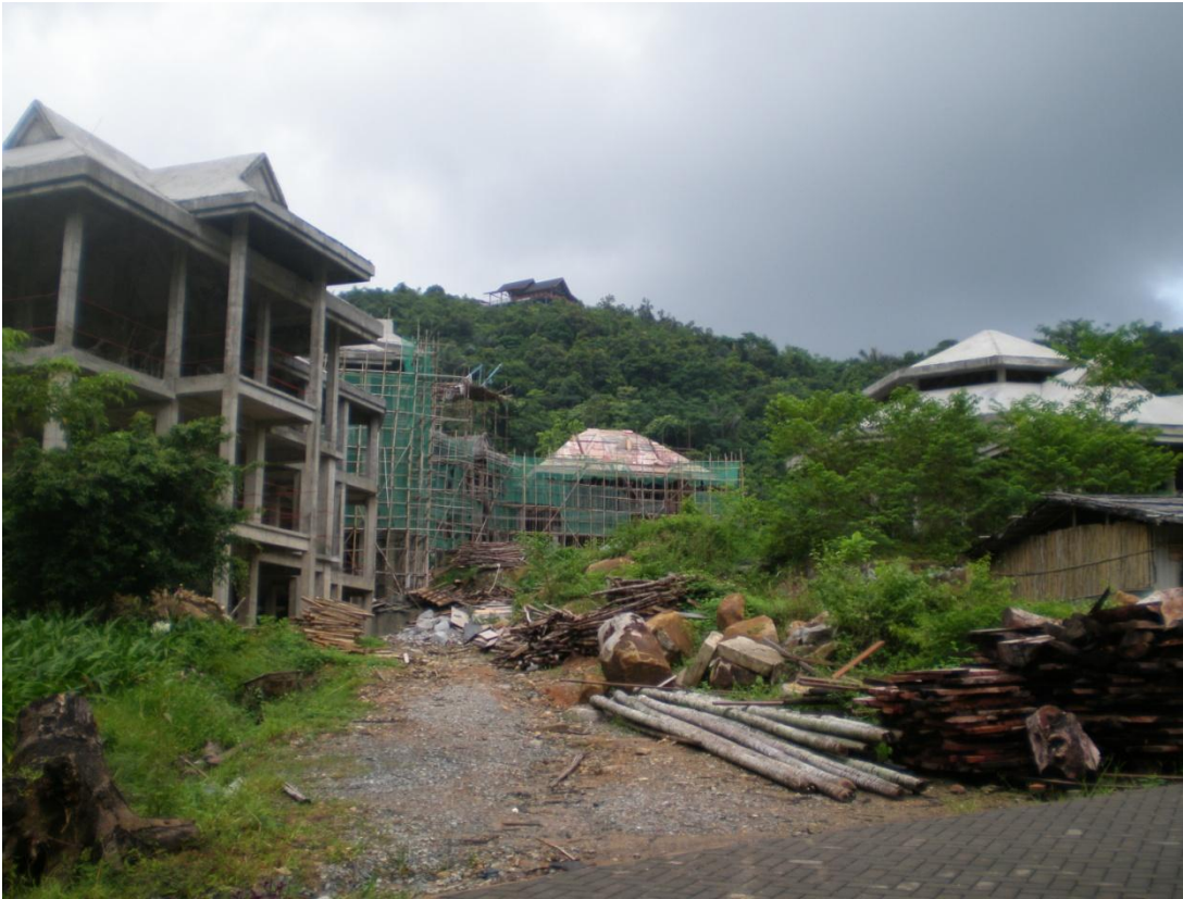
The picture of one construction place (taken by myself)
