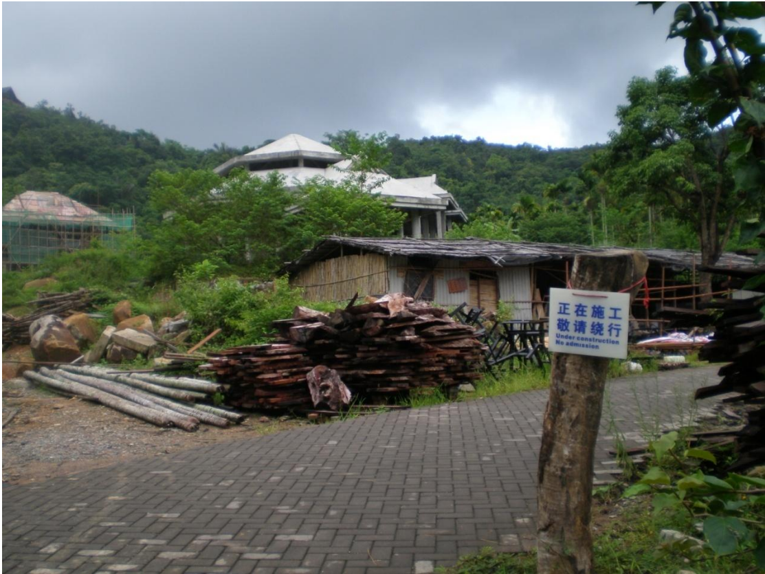
The picture of one construction place (taken by myself)
