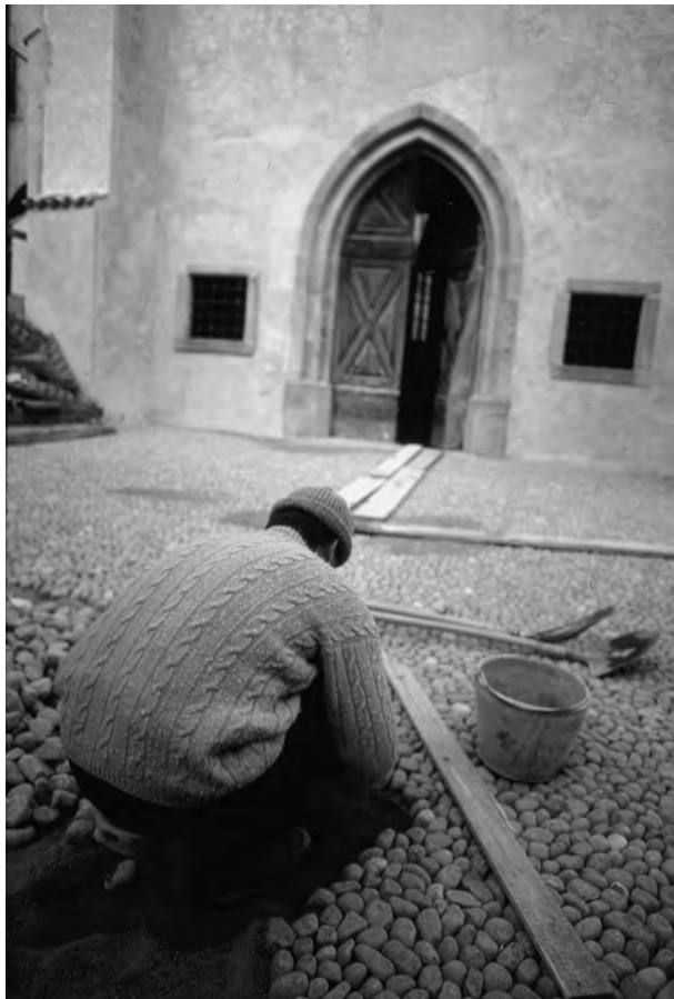
Picture 9. Porphyry stone work in front of San Pietro church. (Photo: Noora Vikman)
