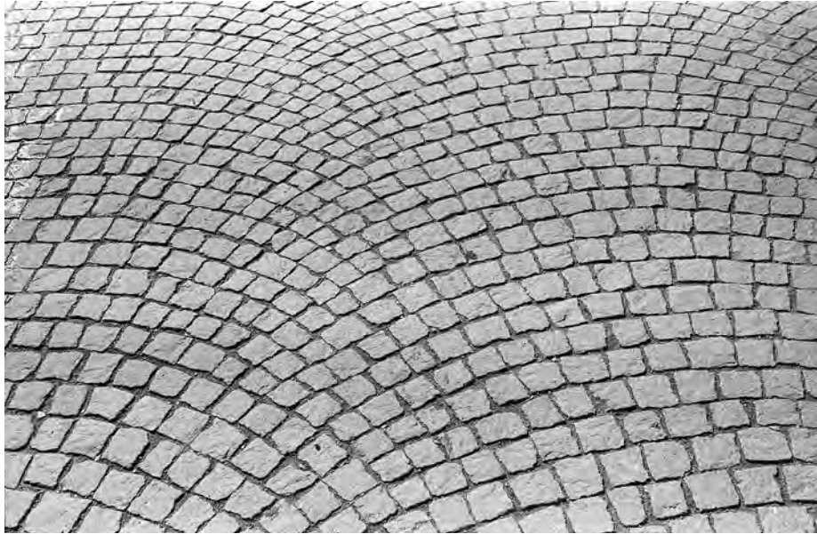
Newly cobbled road in front of the Municipio (Town Hall), Cembra.
