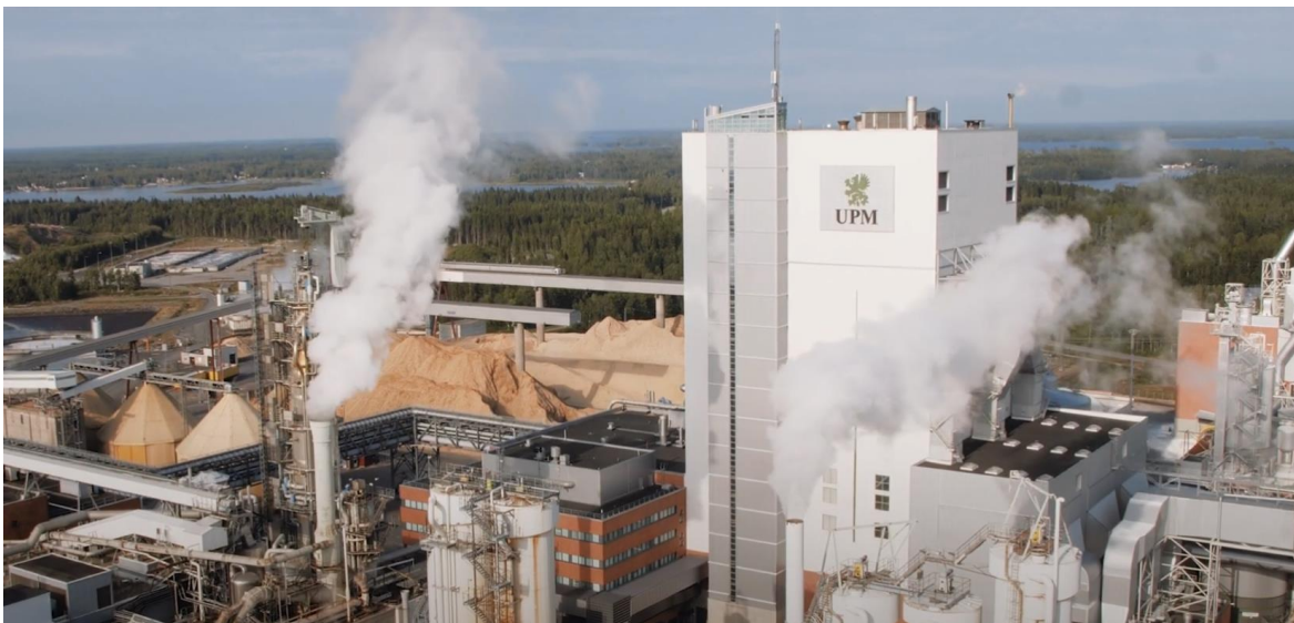
Figur 1. UPM: s cellulosafabrik i Jakobstad. (UPM, 2023).
