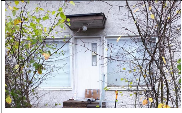
FIGURE 3. Original door and windows with inside shading.
