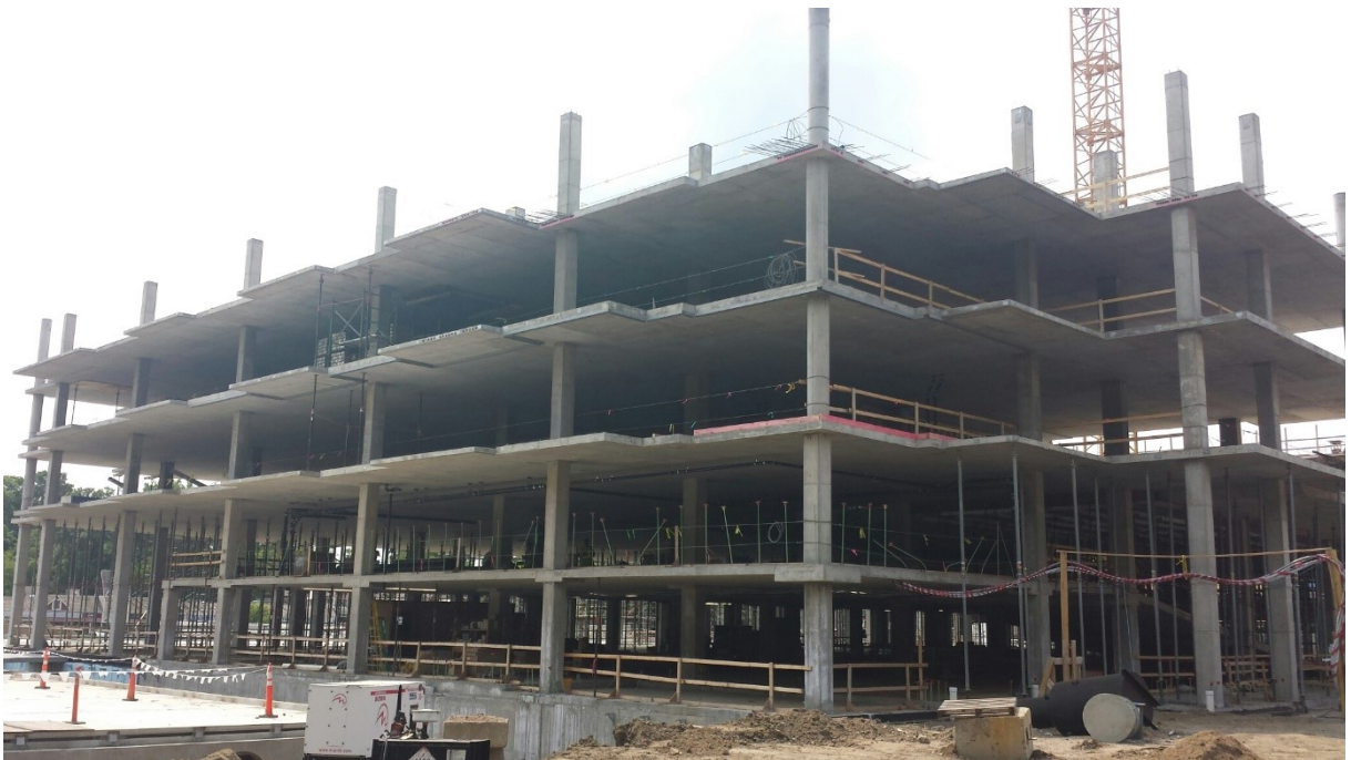
Figure 3.5: Concrete Building Construction (Design Buildings 2020)
