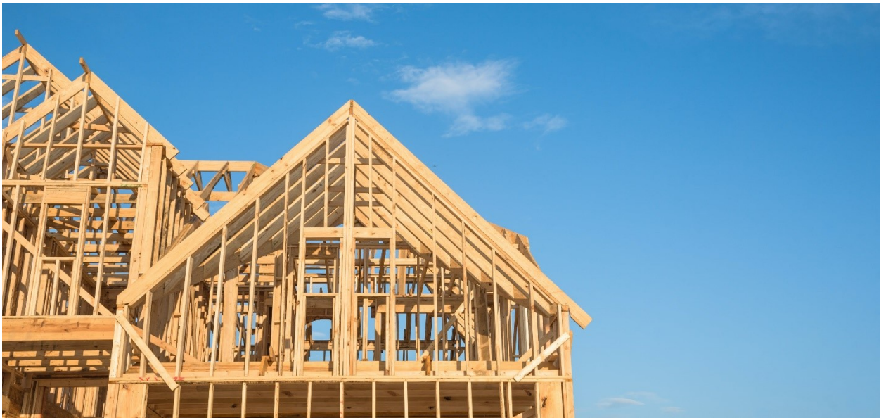
Figure 3.1: Timber structure (Corches, 2019)
