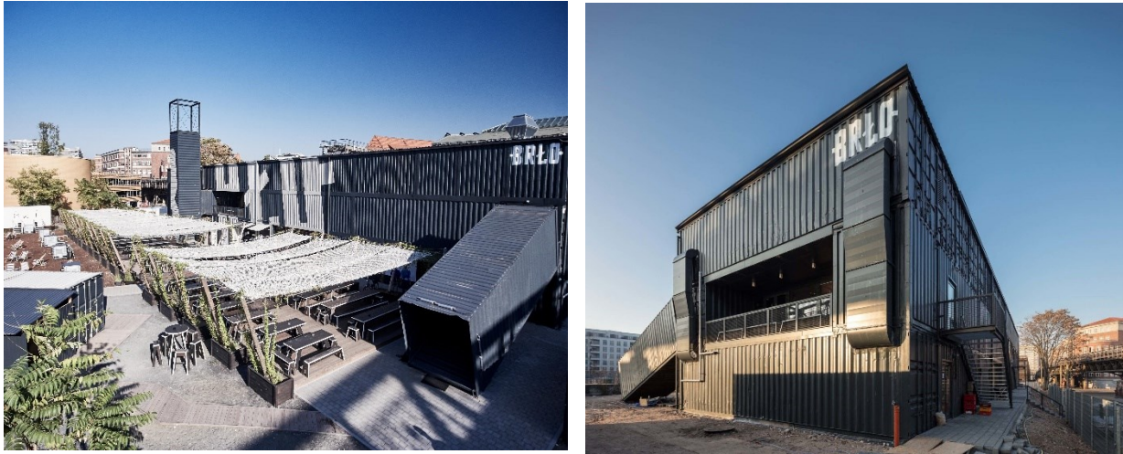
Figure 22: Pictorial view of the vertical, horizontal, and inclined staircase of the BRLO craft beer warehouse (Graft Architects, 2023).
