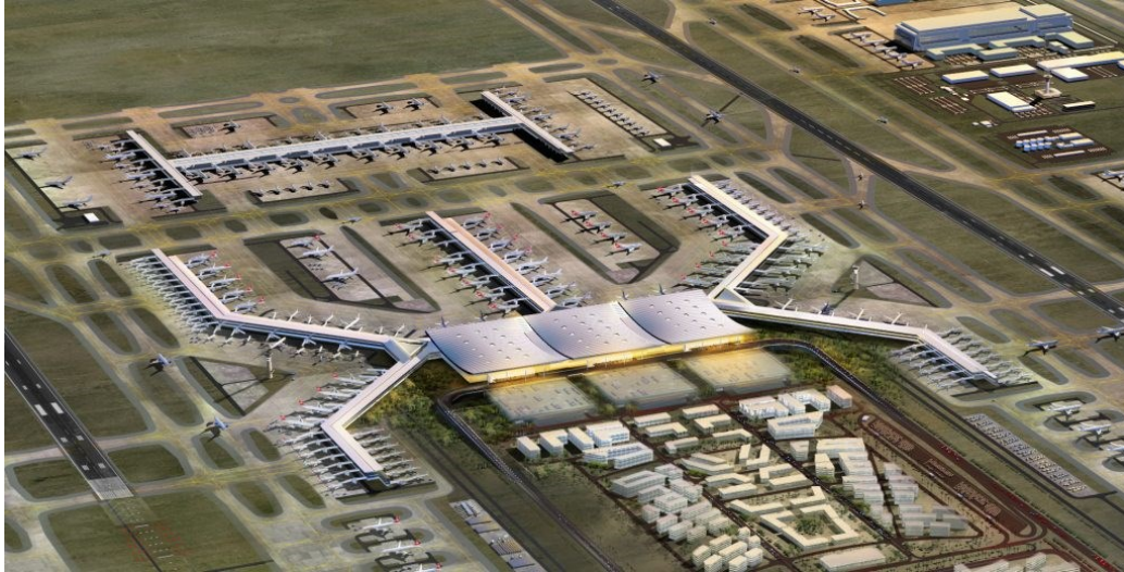
Figure 12: Aerial view of Istanbul Grand Airport, Istanbul, Turkey (BIMCommunity, 2018).
