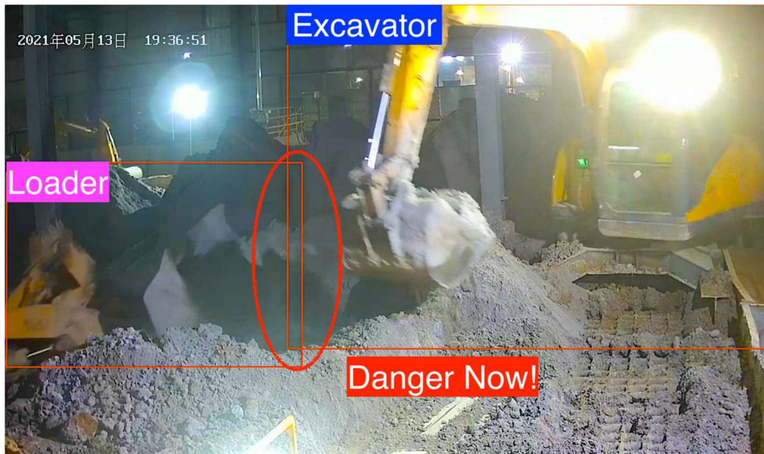
Figure 27 The autonomous excavator and loader potential (S. Zhang & Zhang, 2021, p. 52)
