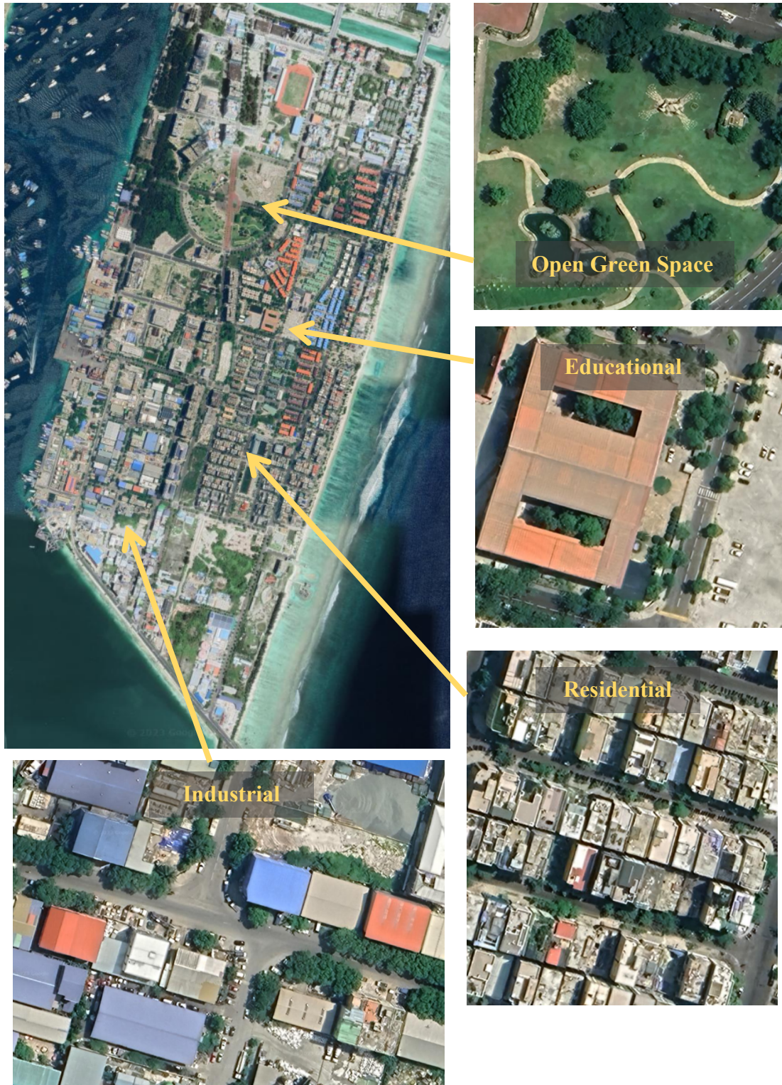
Figure 29: Aerial photos of some land use categories in Hulhumale' phase 1 (Google Earth, 2023)
