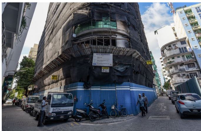
Figure 48: Residential streets in Male' are generally characterized by narrow streets in comparison (Nishaath, 2019)
