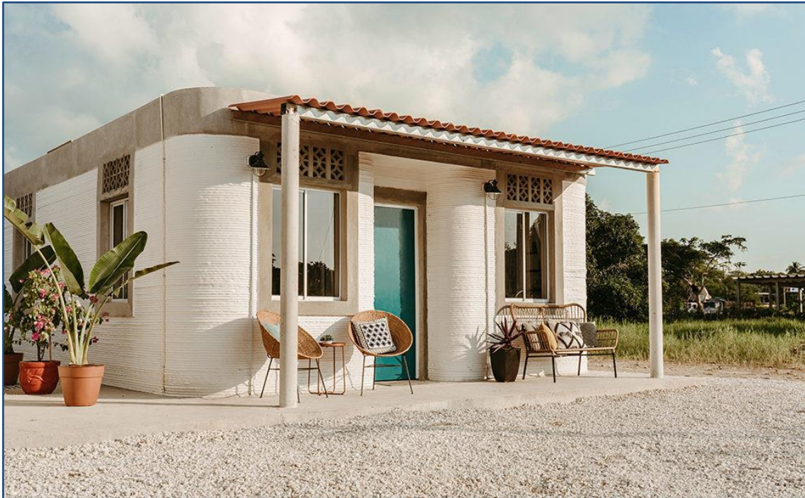
Fig. 29 One of the houses printed in Mexico 36
