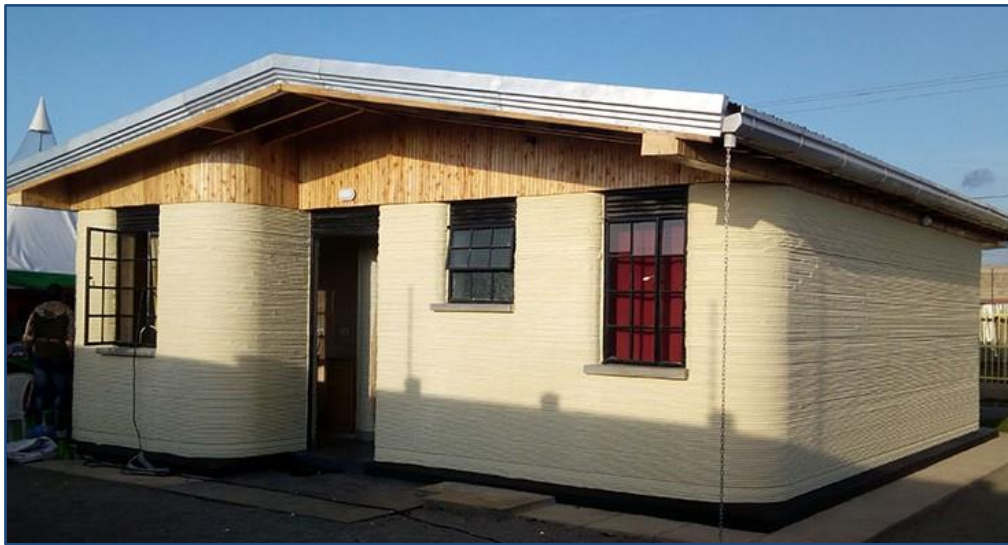
Fig. 27 Tree House No 0. The first 3D printed house in Kenya. Built by 14trees 34
