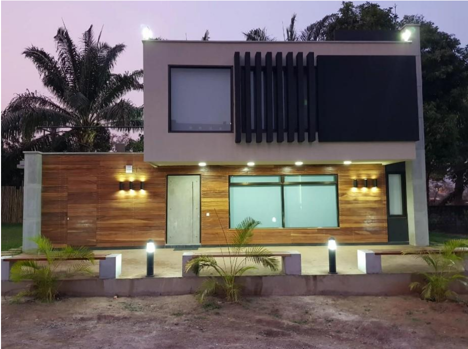
Figure 7: Finished building constructed with shipping container. 7
