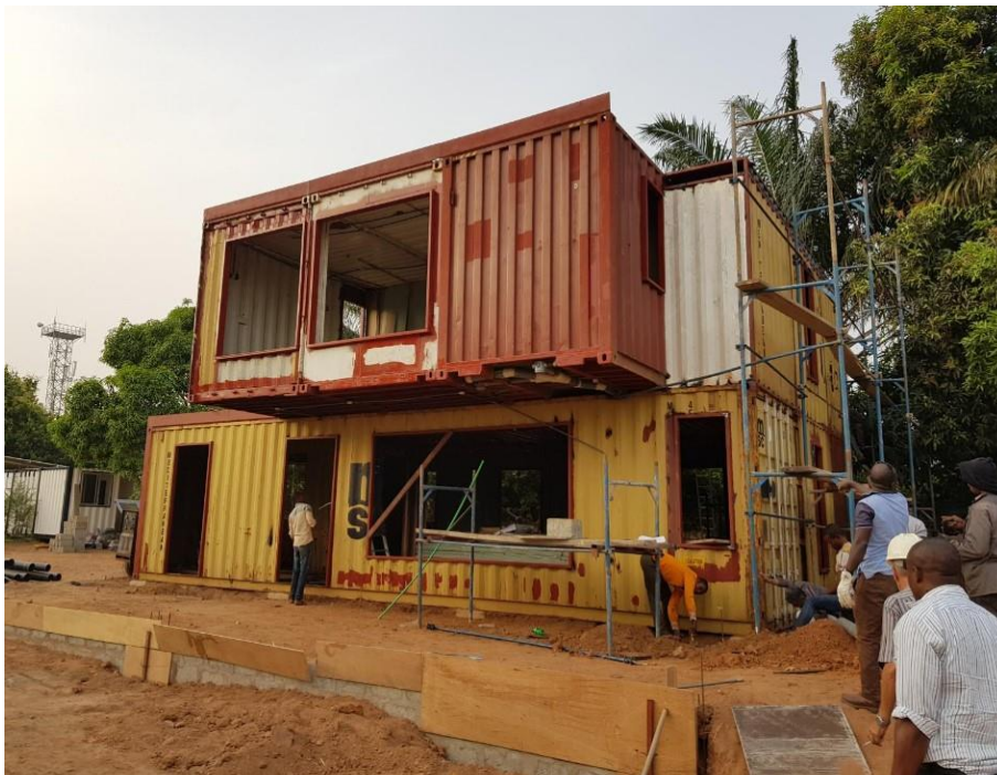
Figure 6: Shipping Container family house under construction 6
