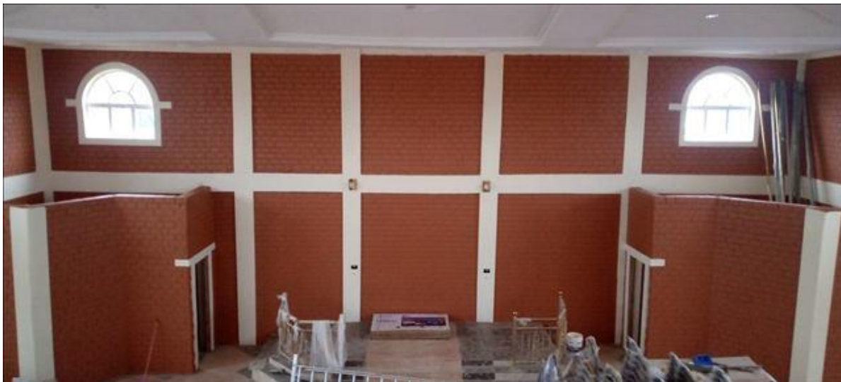
Figure 22: Rendered columns and beams 28
