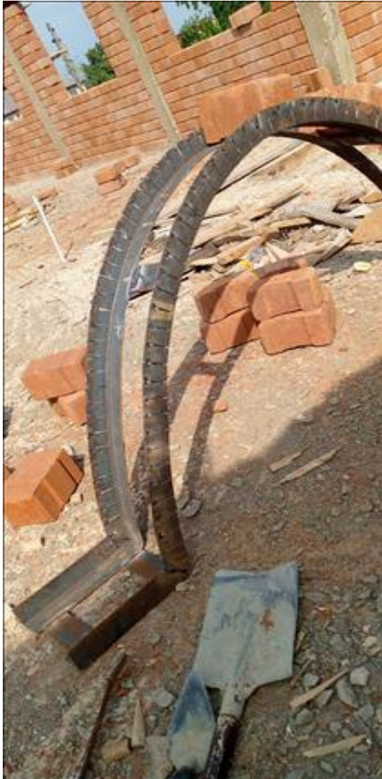
Figure 20: Lintel made with steel 26
