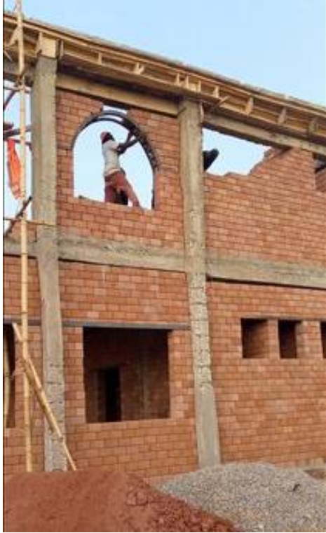
Figure 21: Lintel positioning 27
