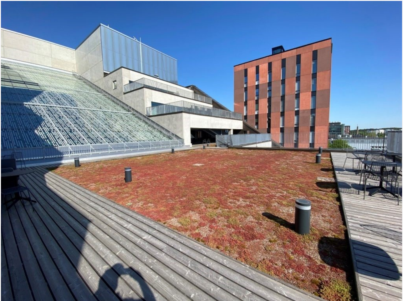
Picture 2. EduCity's green roof of rooftop terrace that was used as a test environment.
