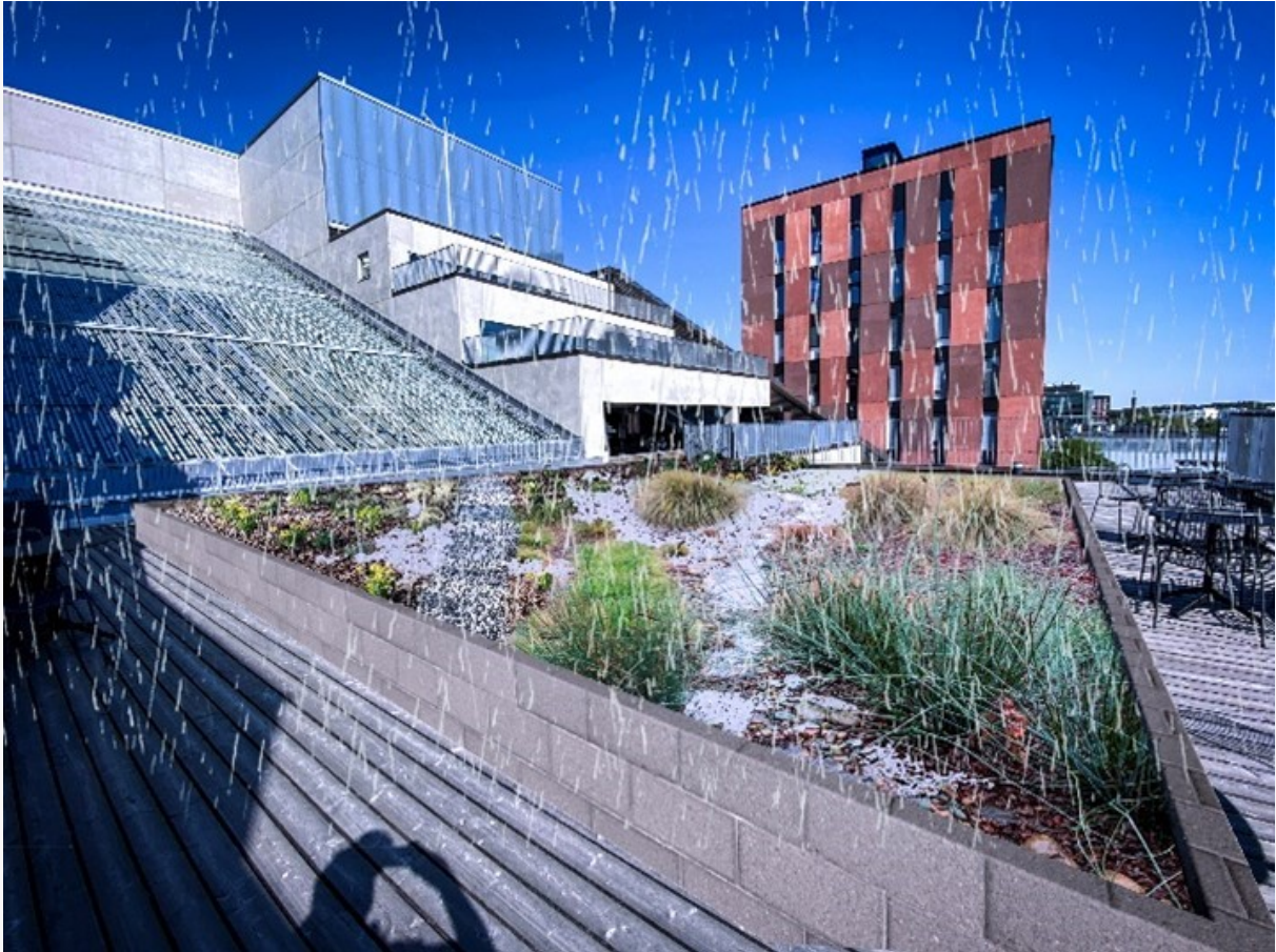
Figures 6 and 7. Visualization of the test site with the designed intensive green roof in dry conditions and during simulated rain.
