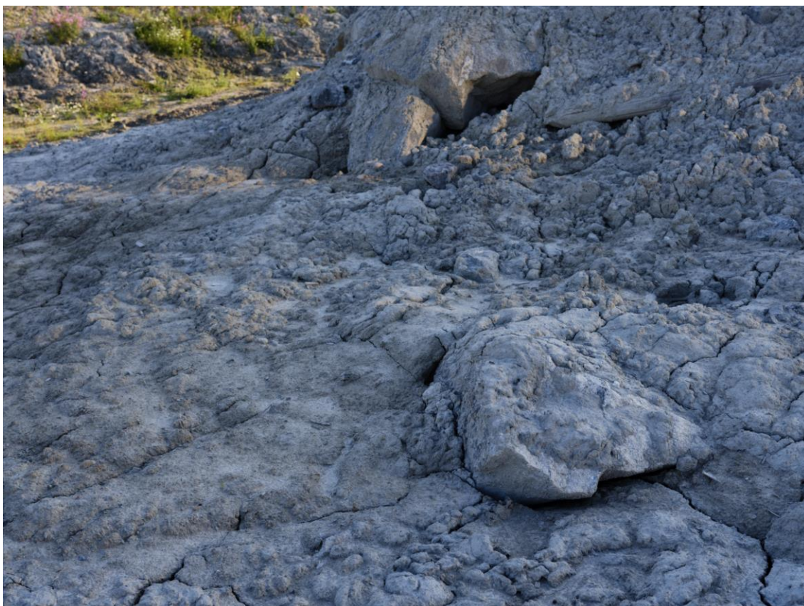
PICTURE 17. Mud at construction site A (2021).
