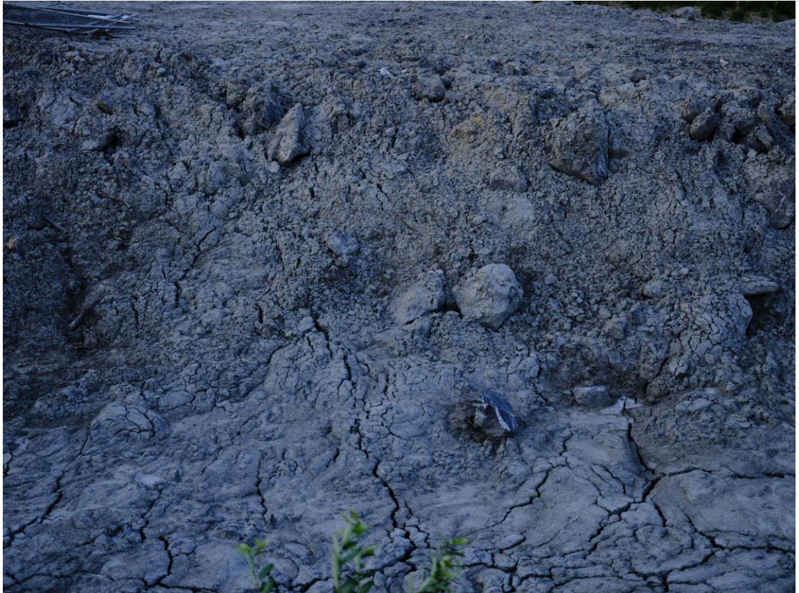
PICTURE 18. Mud at construction site B (2021).
