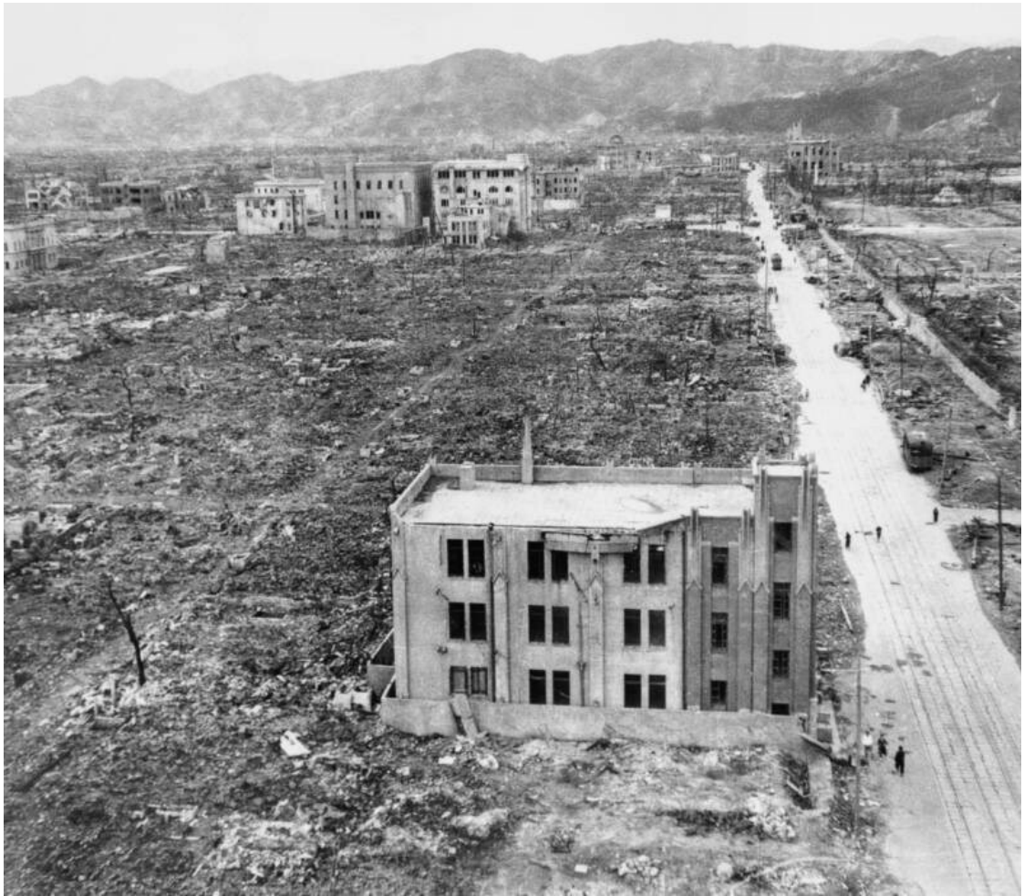
Appendix 4. Buildings reinforced to withstand earthquakes were the only ones still standing after detonation. (Imperial War Museums via Getty Images. https://allthatsinteresting.com/hiroshima-aftermath-pictures#10 .)
