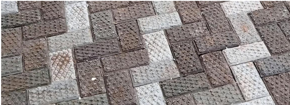
PICTURE 3. Plastic bricks made from recycled waste plastics (Rain Noe, 2021).
