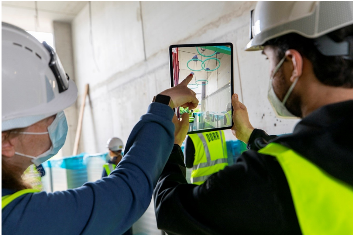
Figure 3. Clarifying the location of lamps using BIM.
