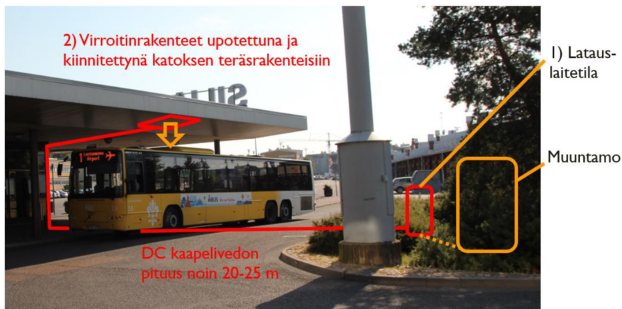
Figure 4. An illustration of the fast charging installation at the Turku harbor, an excerpt from the RFQ documentation provided to the participants in tendering
