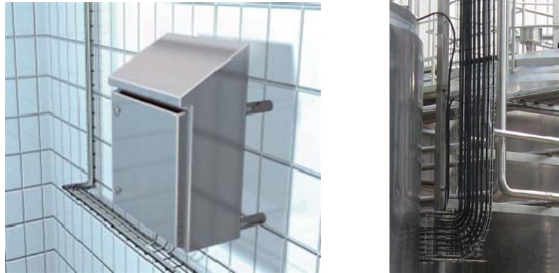
Figure 2: Cleanable arrangements of control cabinet and cabling
