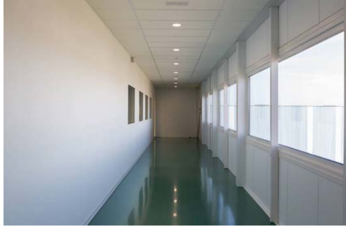
Figure 8: The box in box design with the production zone at the left
