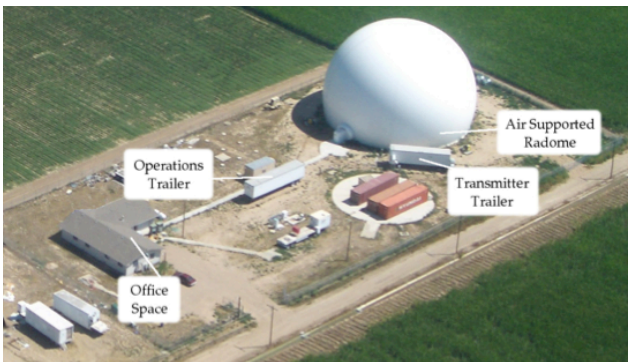
FIGURE I. CSU-CHILL radar facility, with labels indicating major features.
