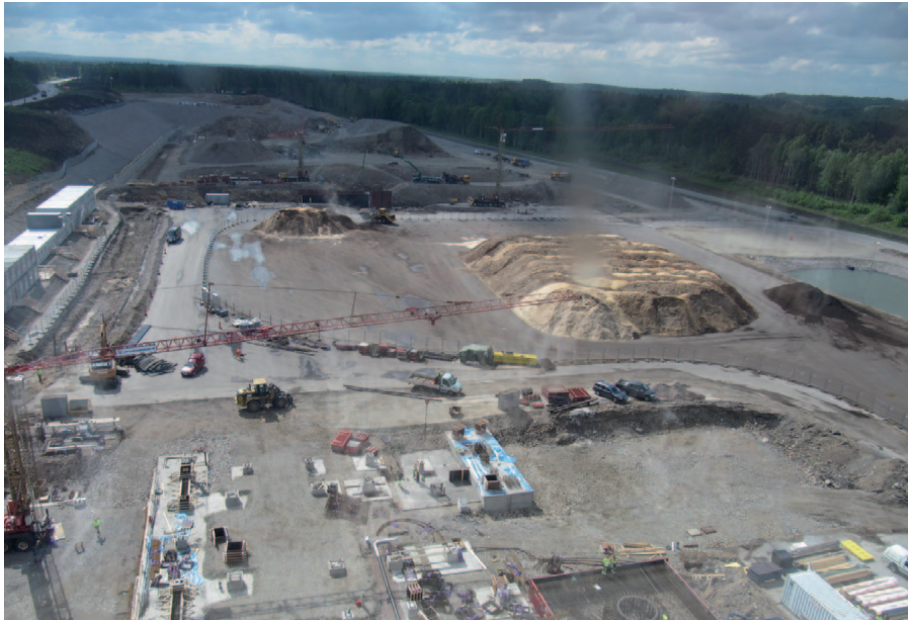
Figure 1. Sandvik 3 is under construction (Photo: Anne Ahtiainen).
