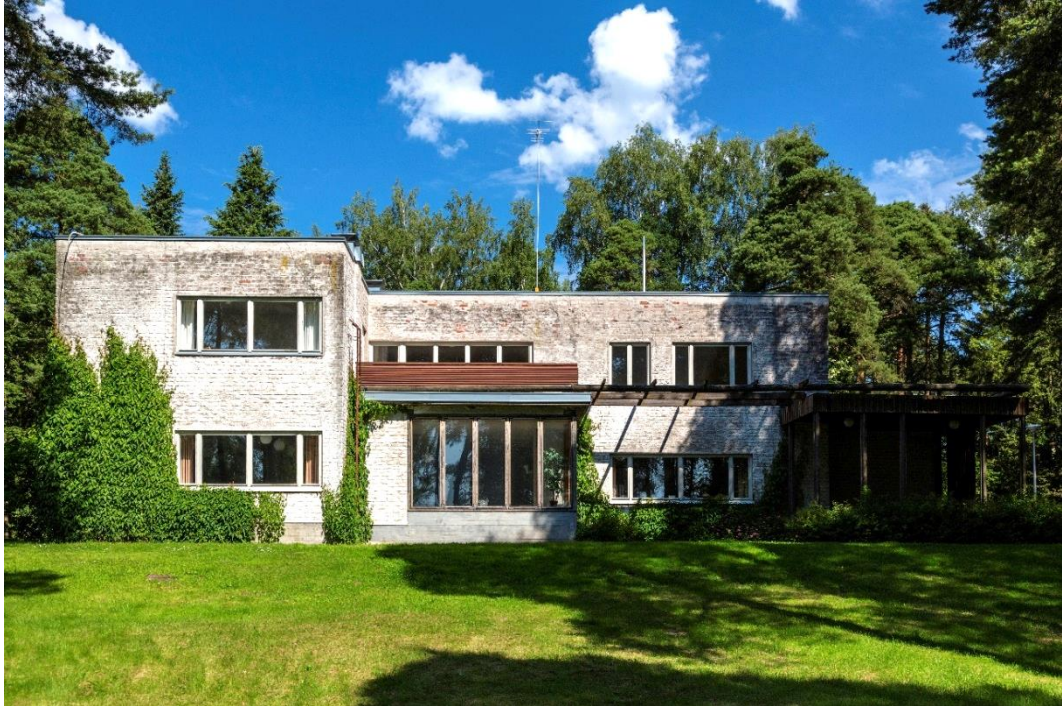
Figure 9: The large windows of Sunila Mill Director's house.
