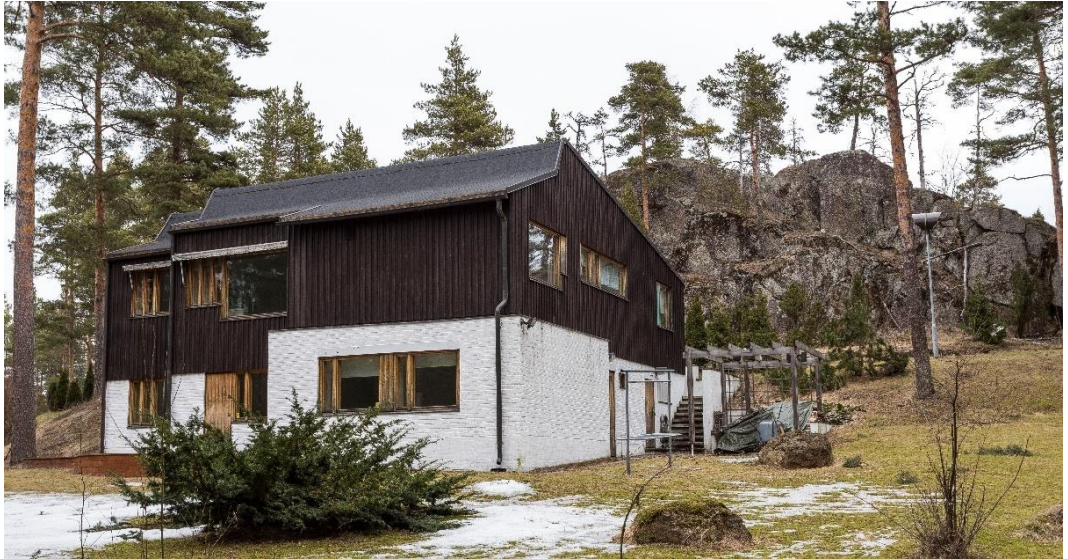
Figure 6: House at Summa blends into the nature of the hill and emulates the form of the rocky outcrop behind.
