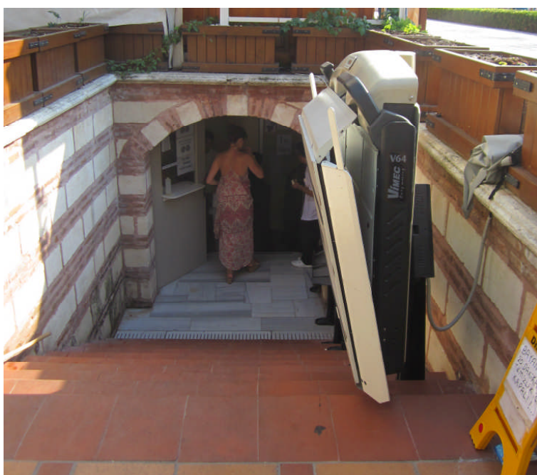
Image 11: Wheelchair elevator to the public toilet
