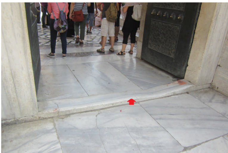
Image 36: The 8 cm treshold after the ramp
