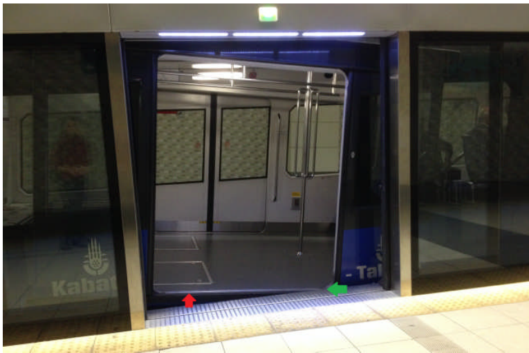
Image 4: Platform and funicular trains' floor level difference
