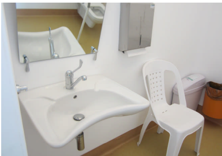
Image 19: Sink and chair in the accessible toilet
