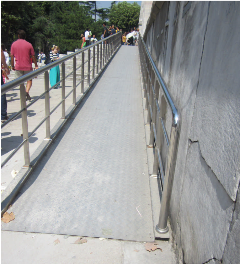
Image 35: The ramp to the courtyard
