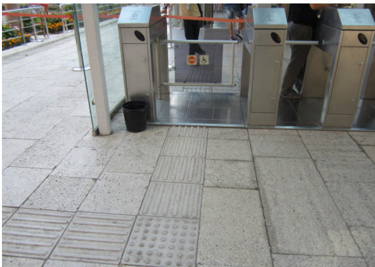
Image 23: Ticket gate for wheelchair and markings for blind
