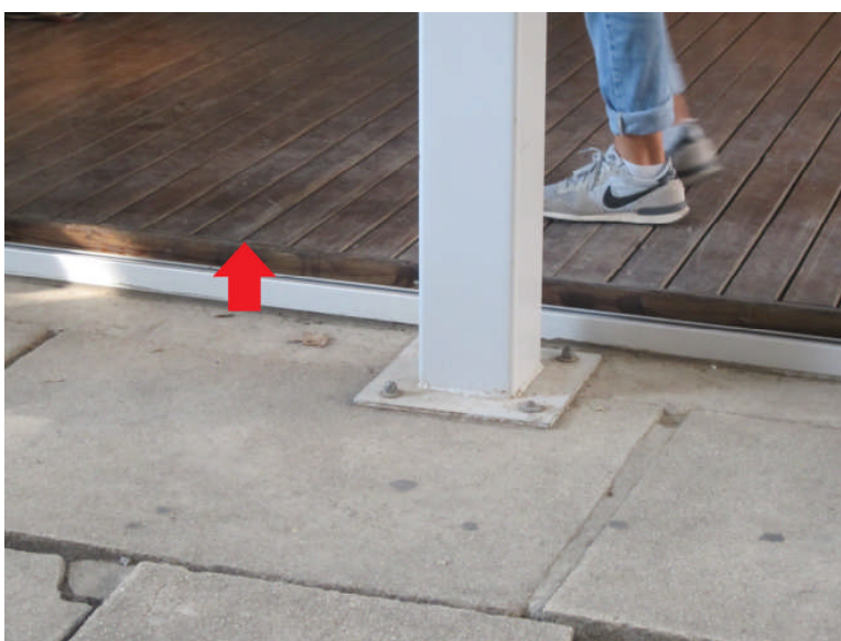
Image 31: Threshold to the cafes service counter
