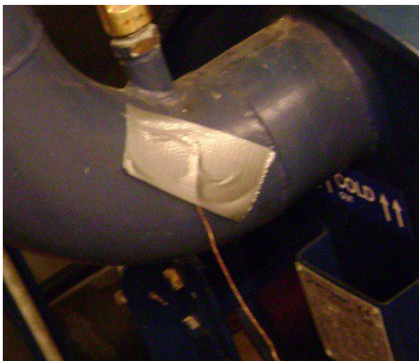
Figure 5: Bad sensor placement; source: KyAMK EnergyLab
