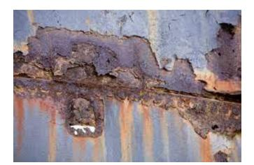
Figure 7: Selective Corrosion (Moriber, 2020)
