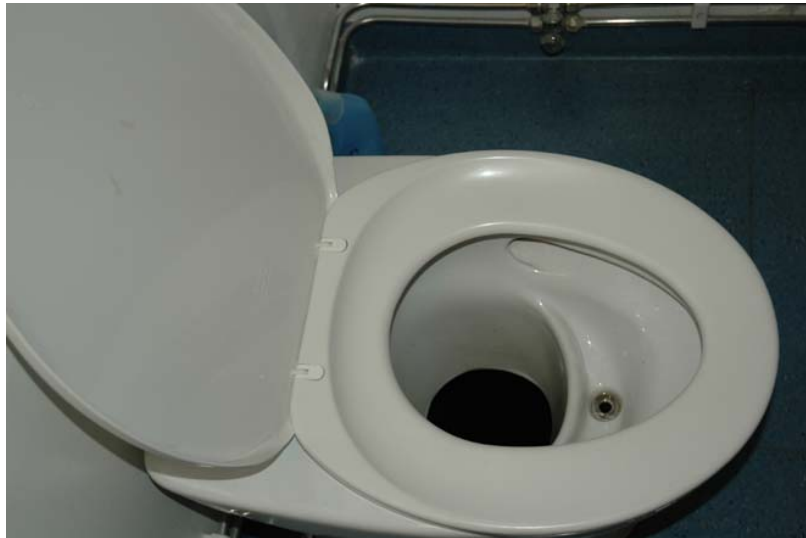
Figure 3. Example of a urine-diverting dry toilet seat. The urine is diverted to the front of the seat (right) and faeces with toilet paper falls freely without water from the back (left). (photo: Outi Palttala)
