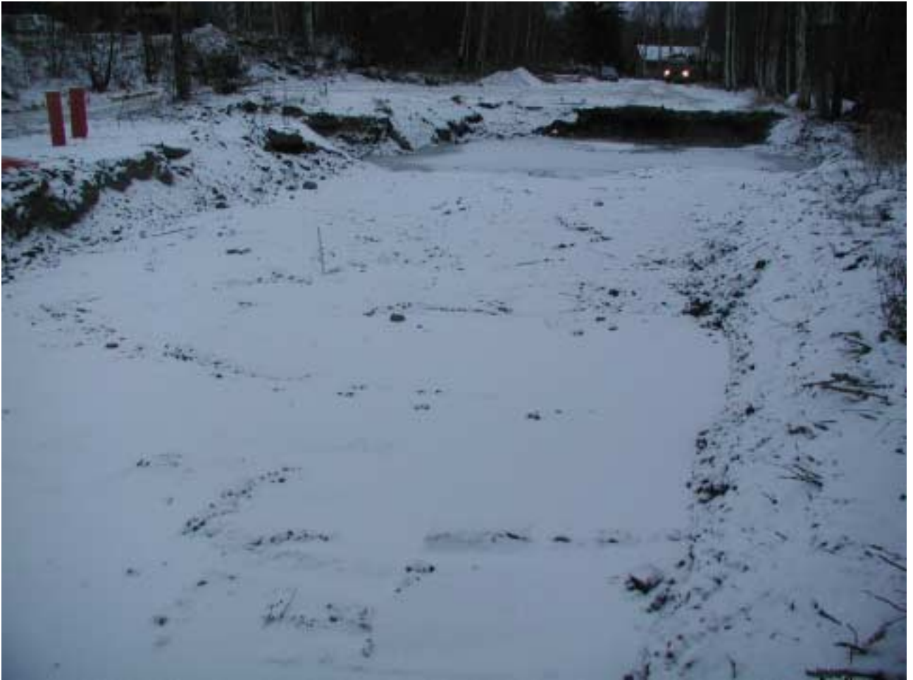
Figure 5: Warehouse area. Orientation east.
