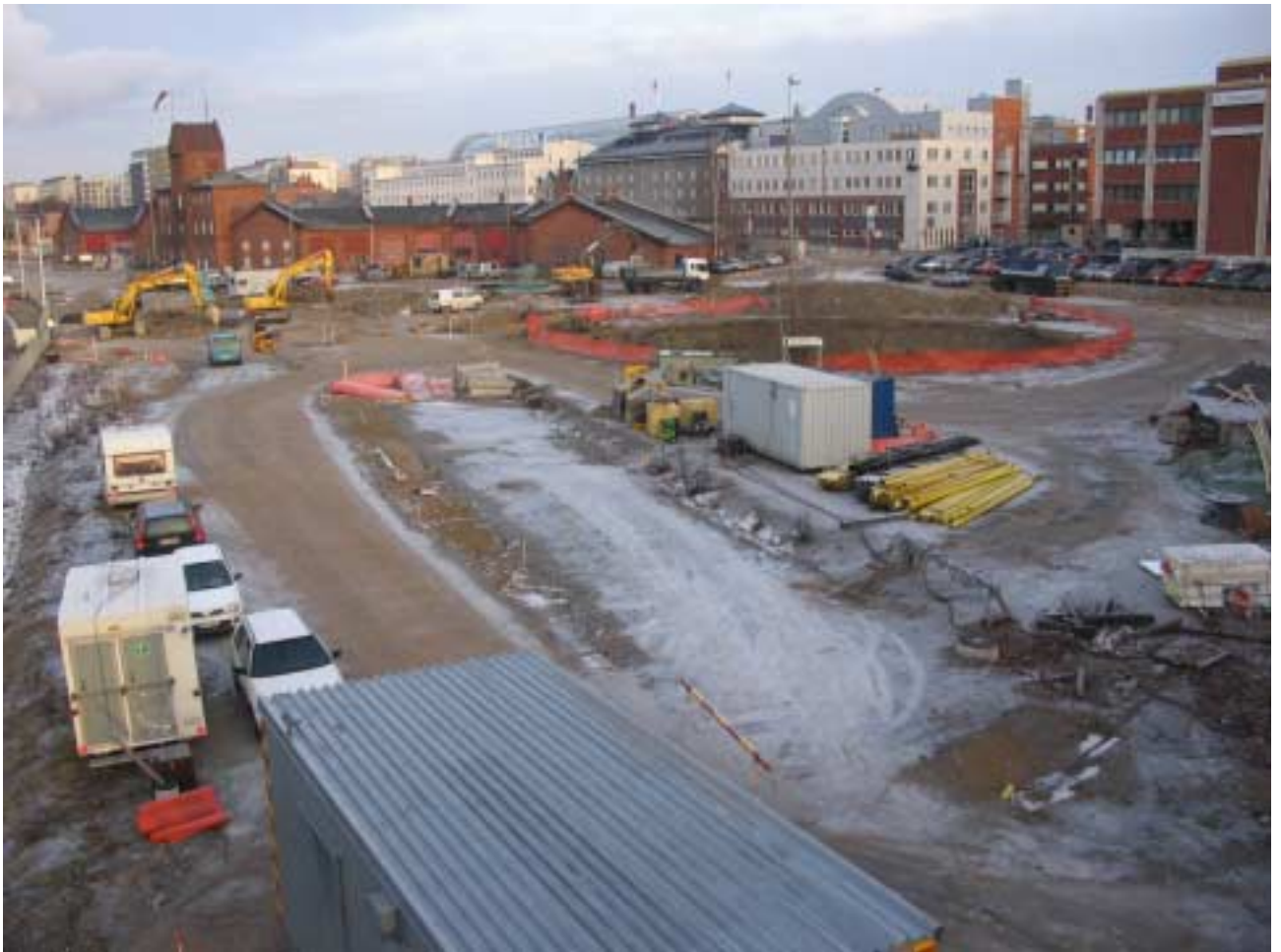
Figure 6: Ratapihankatu renovation in process. Orientation north.
