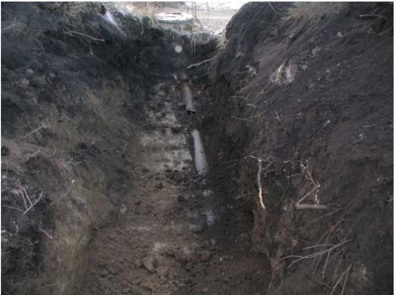
Figure 3: Rainwater drainpipe. Orientation: South.
